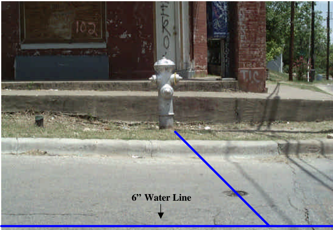
Figure 4 – Fire hydrant at Tenth Street and Cliff Street.
