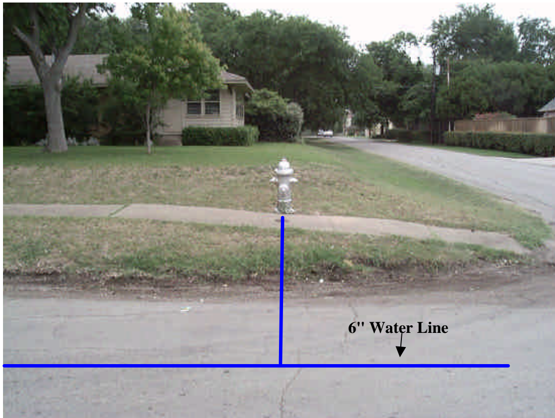
Figure 3 – Looking north at fire hydrant at northwest corner of Lakehurst Avenue and Thackery Street.
