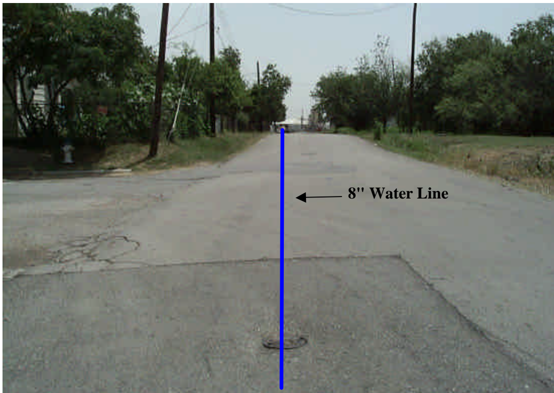
Figure 2 – Looking east across Iroquois Street down Fitchburg Street.
