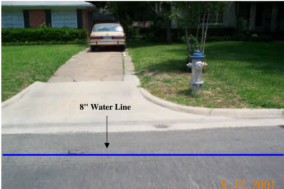
Figure 6 – Looking north from Del Norte at hydrant ? 1,000 ft from Edgemere Road.
