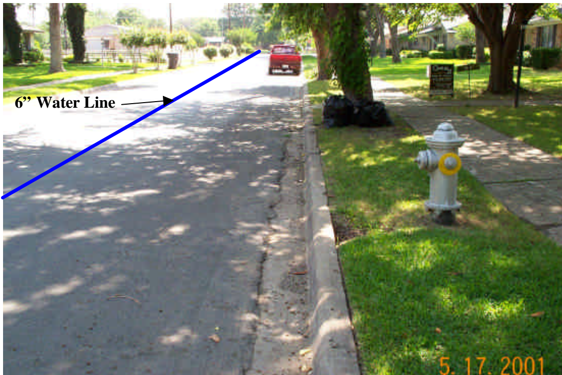
Figure 3 – Looking east near hydrant down Talisman Drive.
