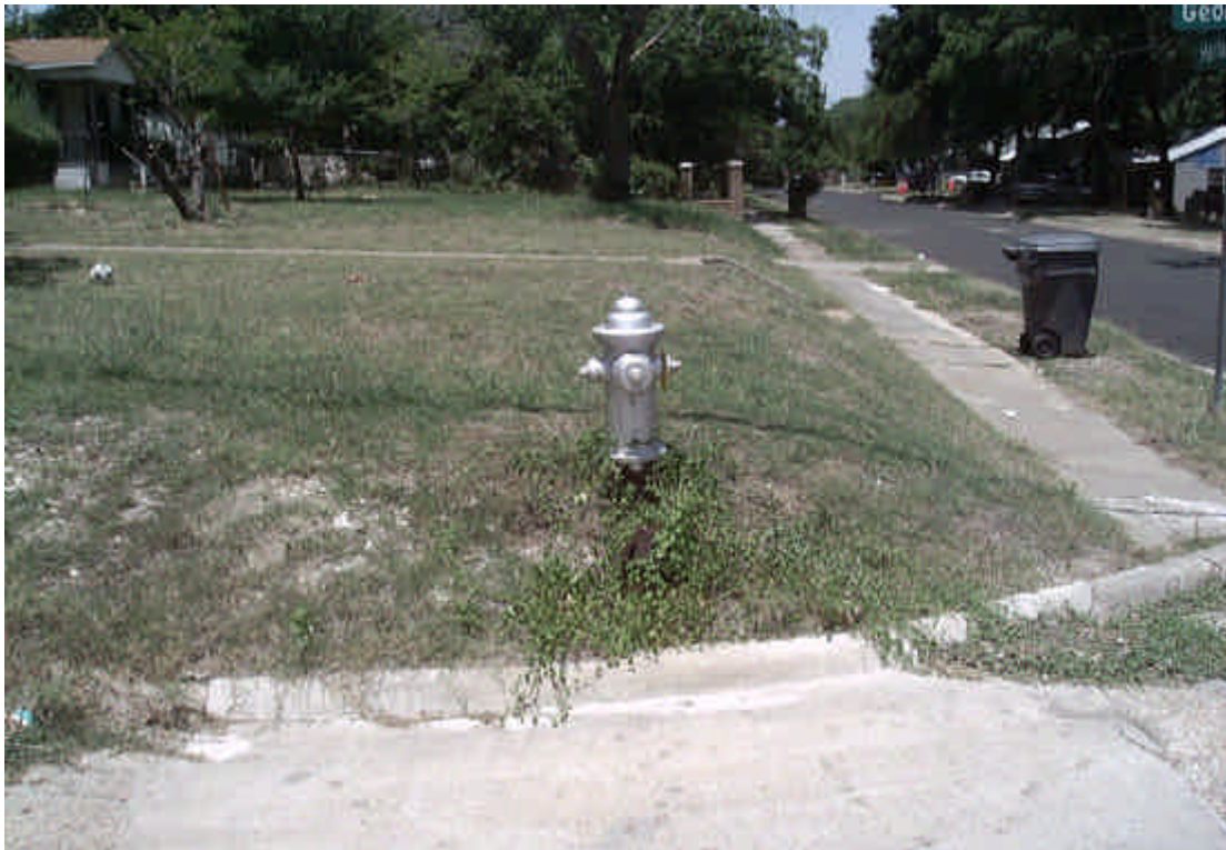
Figure 5 – Looking north at fire hydrant at northwest corner of Harlandale Avenue and Georgia Avenue.
