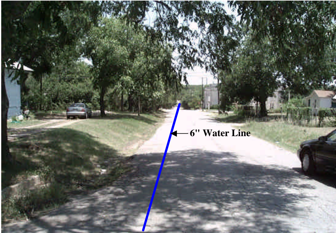
Figure 1 – Looking east at Georgia Avenue from Idaho Street.
