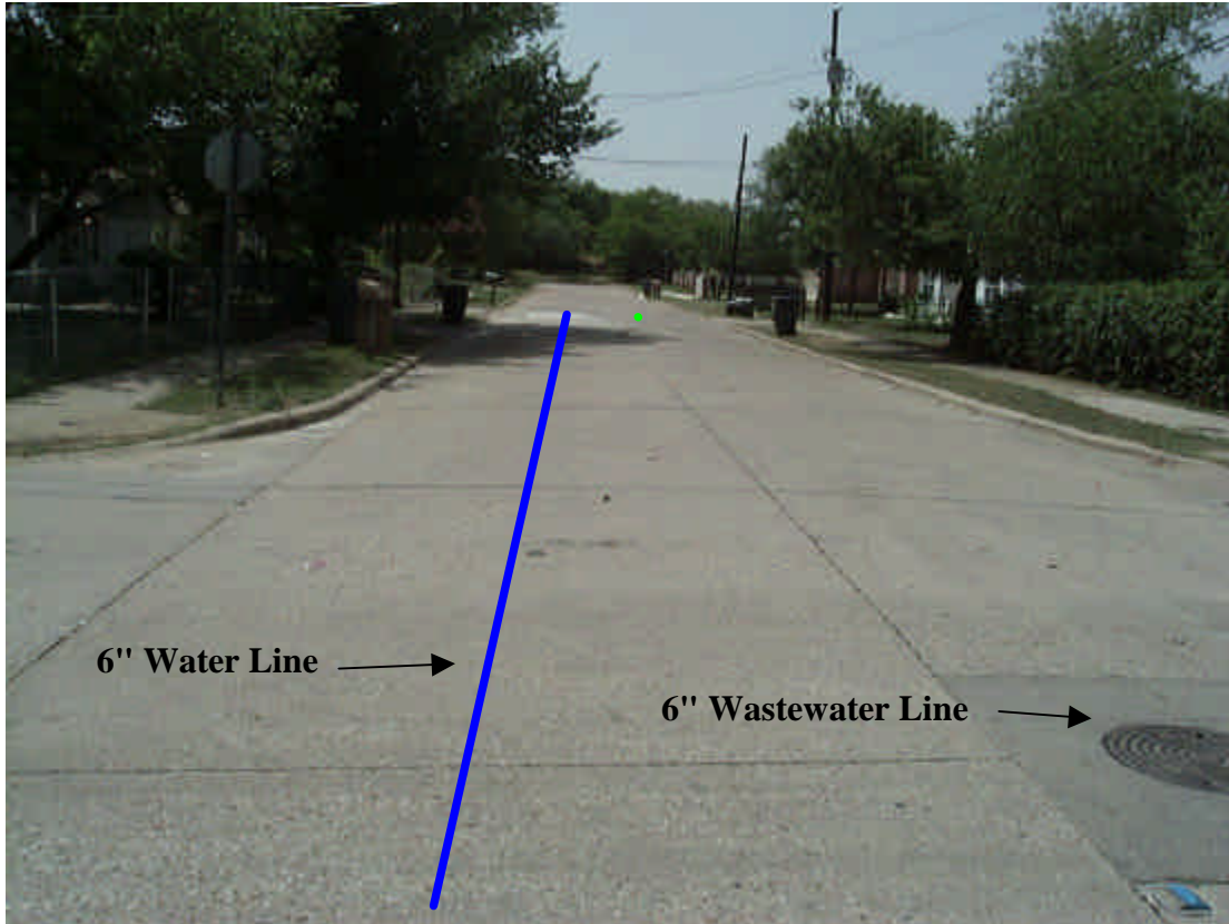
Figure 1 – Looking south from Fitchburg Street down Clymer Street.
