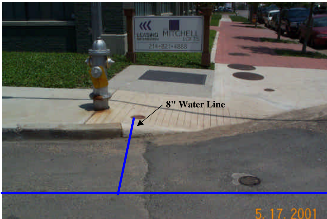
Figure 2 – Looking east at hydrant on northeast corner of Commerce Street and Benson Street.
