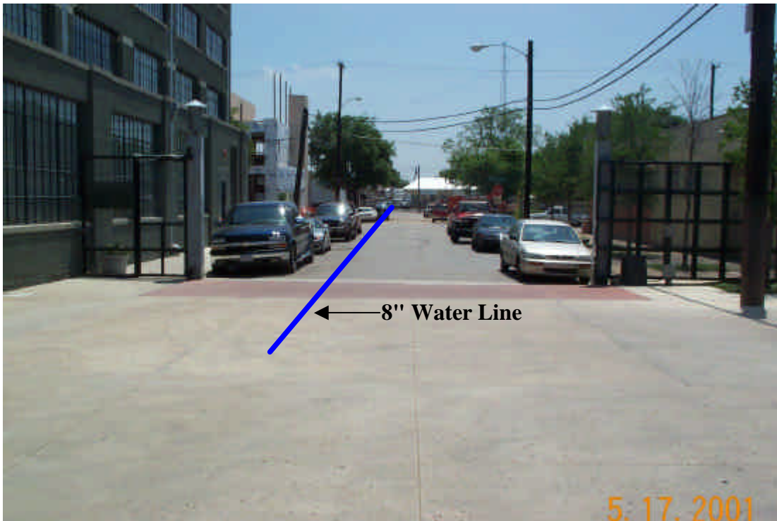
Figure 4 – Looking south from apartment walkway down Benson Street.
