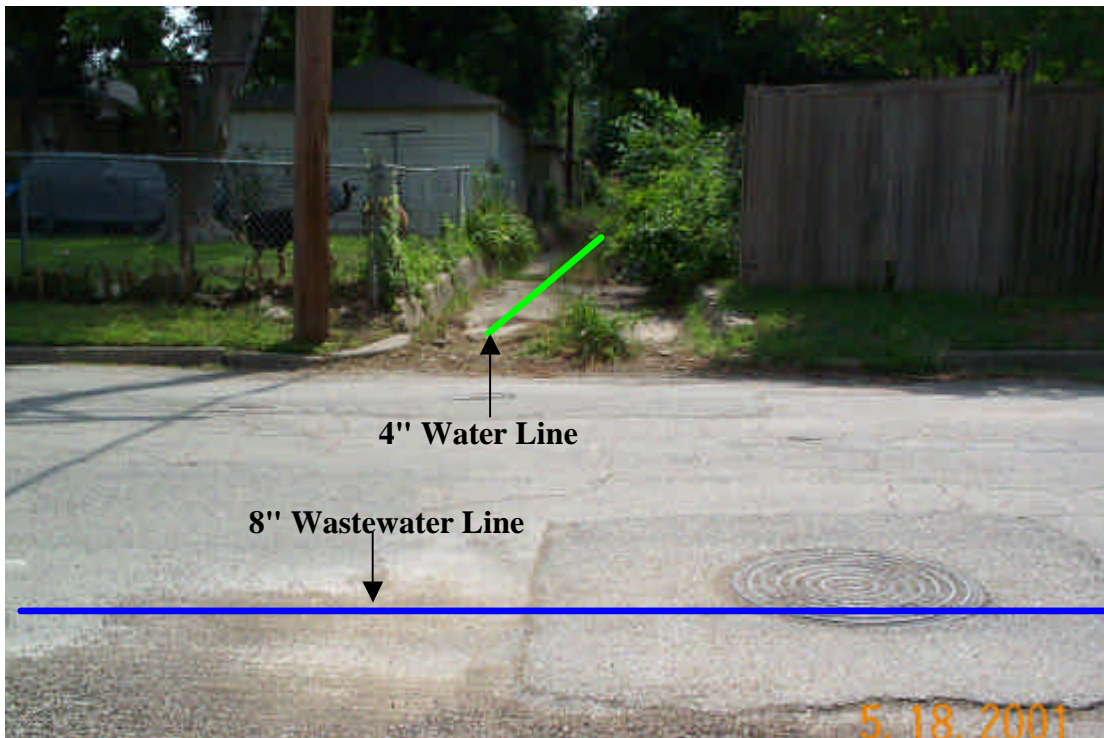
Figure 8 - Looking east from alley between Martel Avenue and Longview Street.
