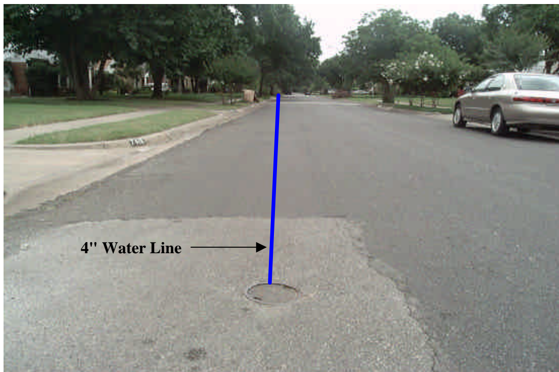
Figure 2 – Looking south at the water valve near the corner of Locksley Avenue and Callet Street.
