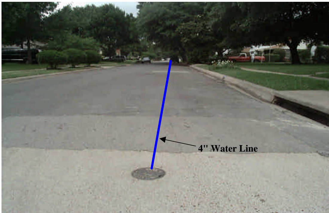
Figure 1 – Looking north at the water valve near the corner of University Boulevard and Callet Street.
